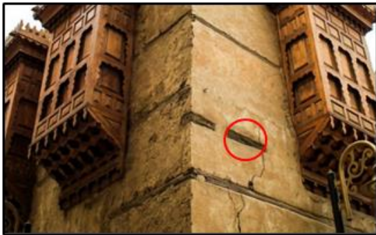
Figure 15. Wood Beams of Historical Jeddah Buildings. (Source: Author, 2024)
